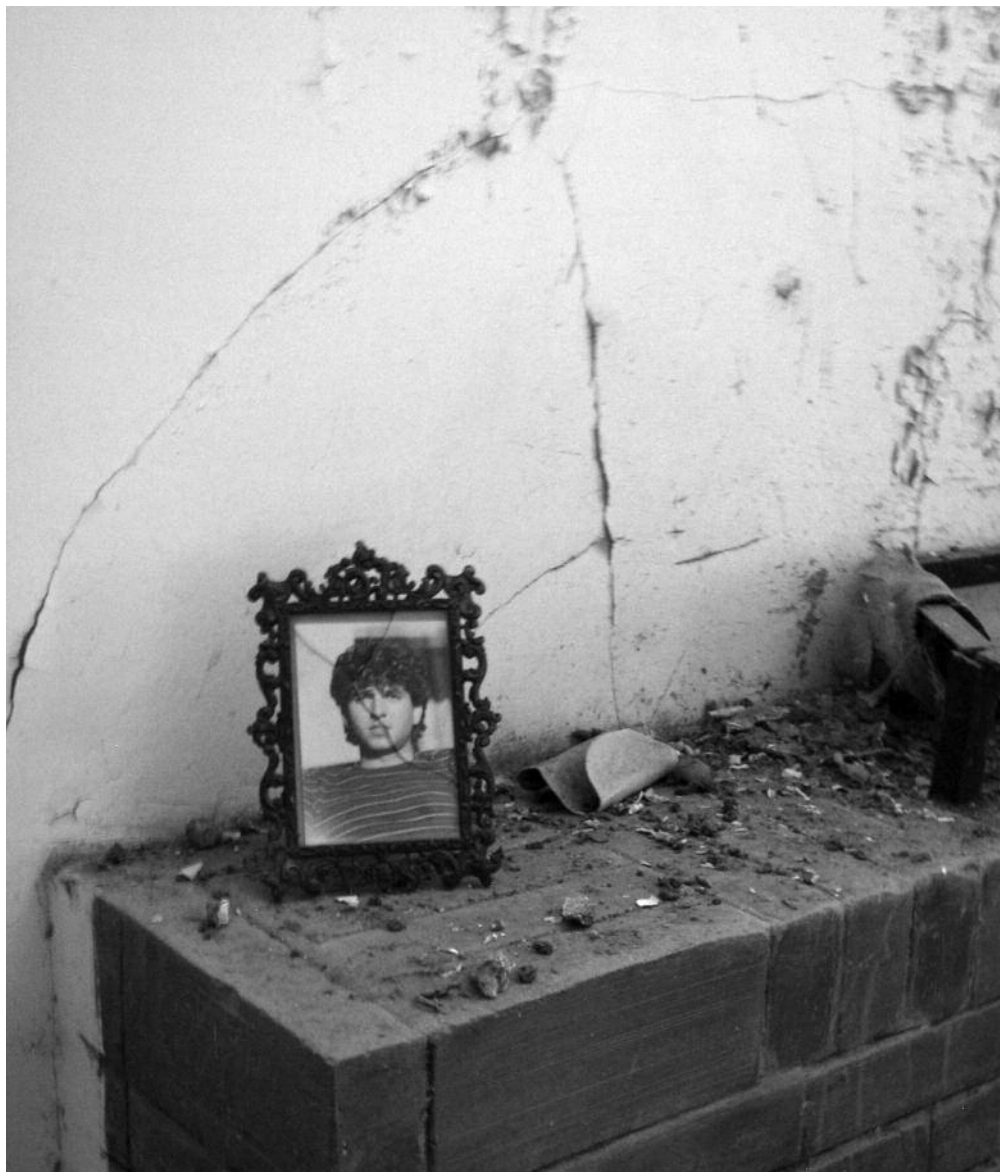
Image 10: Abandoned house in north Nicosia
